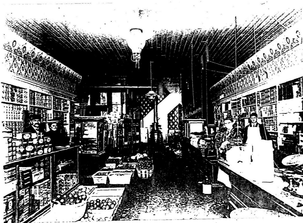
LAMB GROCERY (1910) 101 WEST MICHIGAN AVENUE FORMERLY, KING GROCERY
