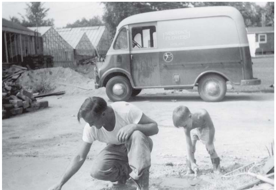
1954 - Austin and Dennis cementing the driveway at the greenhouses on Lowell.
