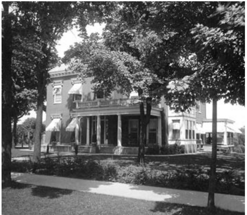
The Quirk residence prior to the addition in 1927 of the extensive theatre arts and circus library.
