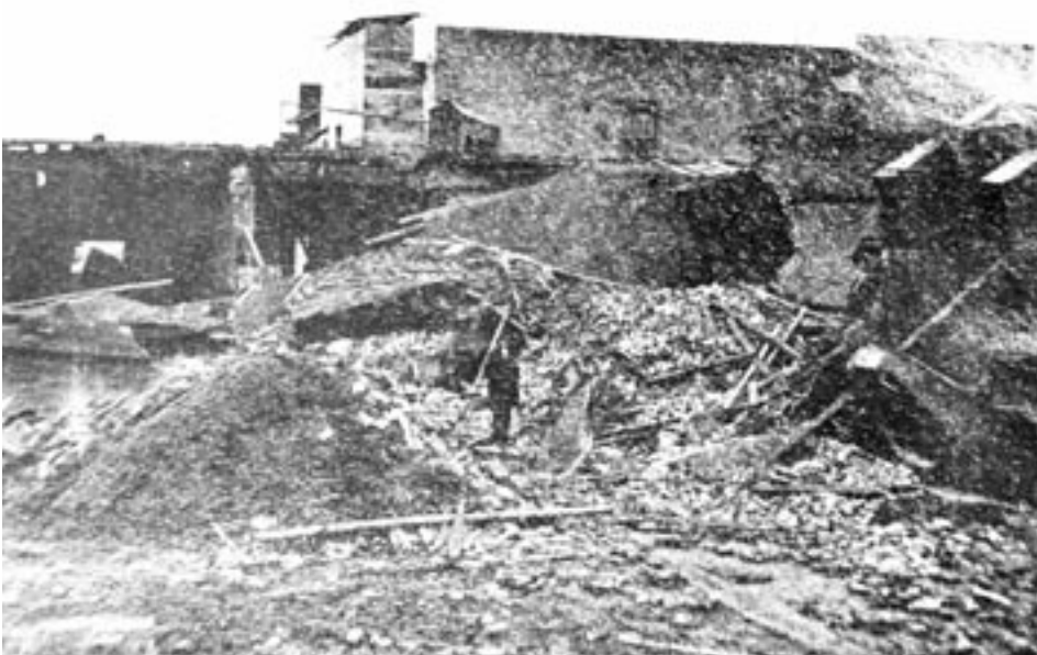
Damage to the Cornwell Mill after the 1876 boiler explosion.
