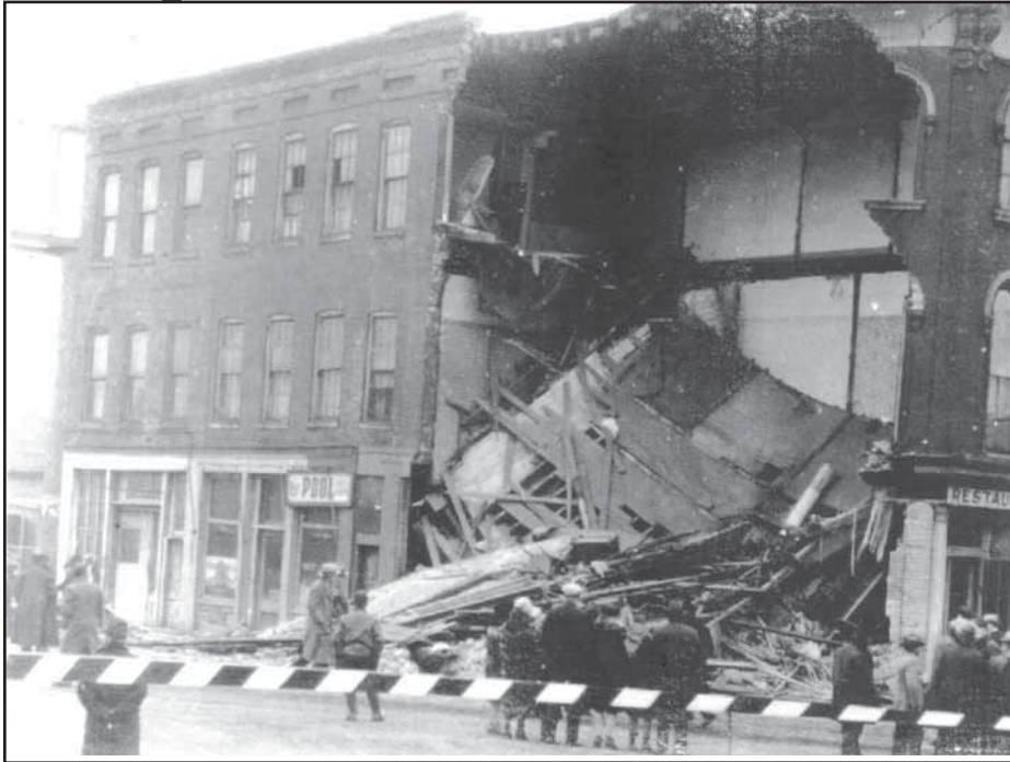
A rare photo of the damage to the Cadwell Building (now the Sidetrack Bar and Grill) from the train wreck on January 21, 1929
