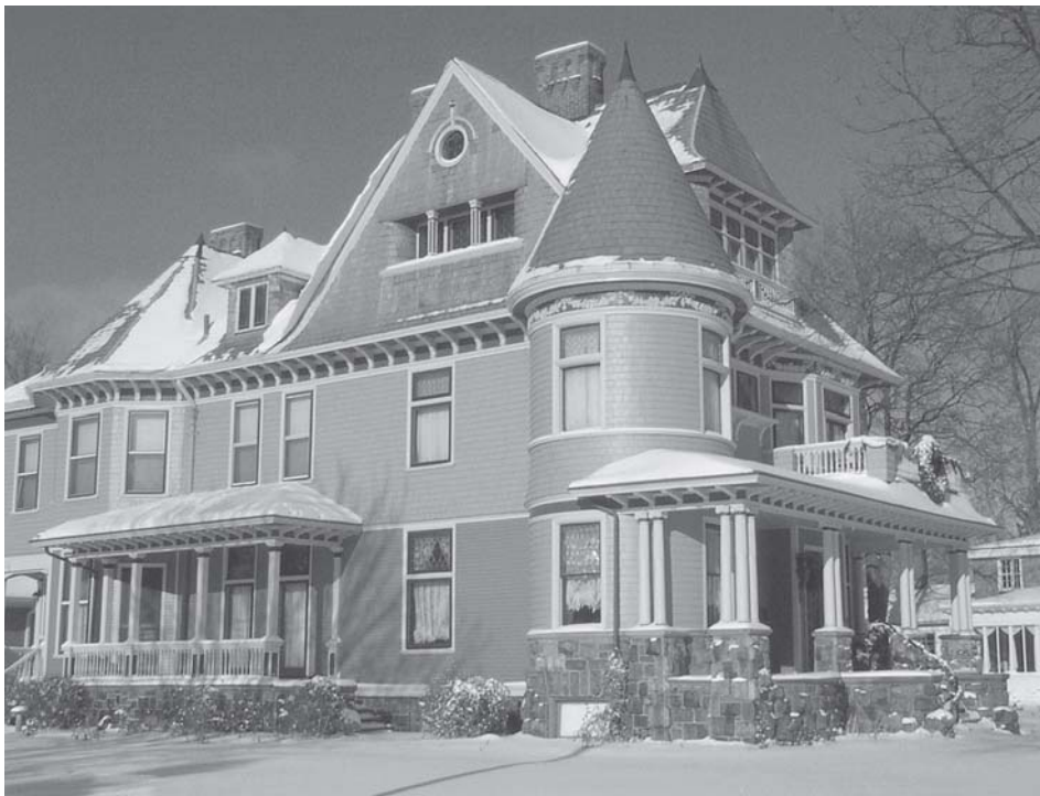
Exterior of house exhibits late Victorian period features.
