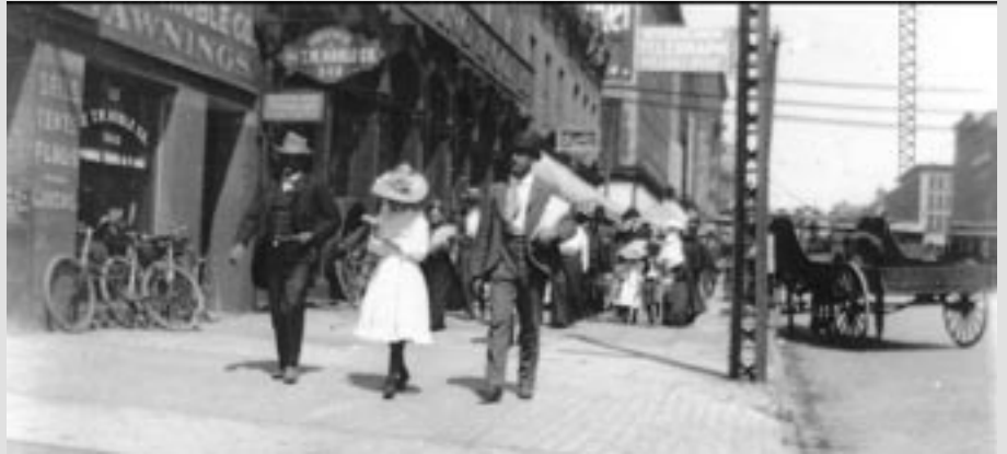
Light towers in the City of Detroit included "arm lamps" (to right of walkers) at major intersections and "moon towers" (background at right) in residential wards.
