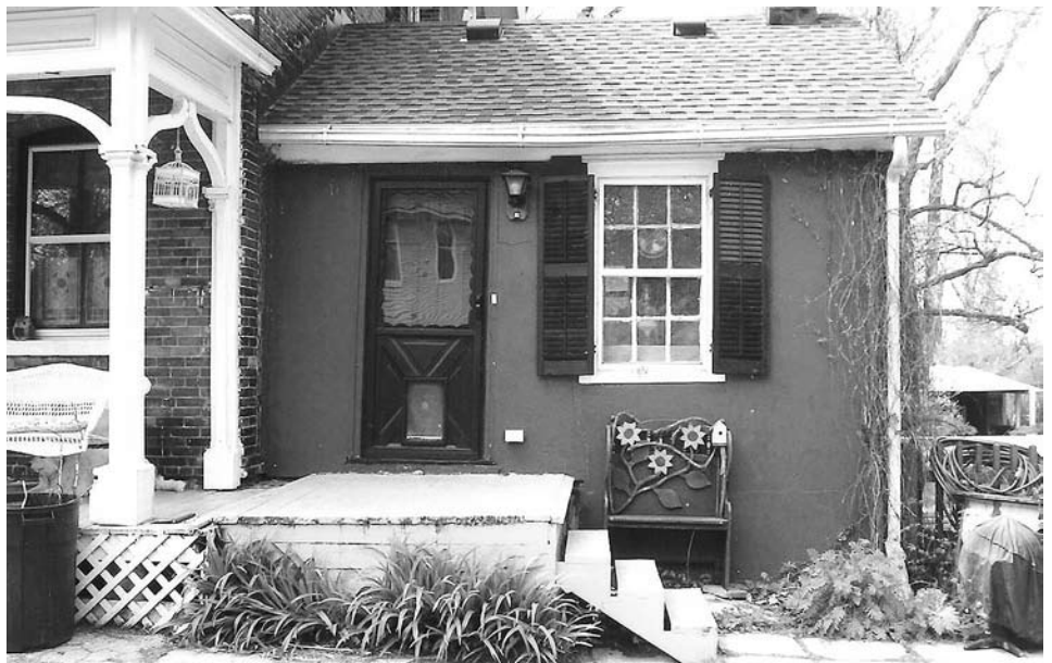
Photo shows the current kitchen portion of the Swaine house that is believed to have originally been a part of the Peck house.
