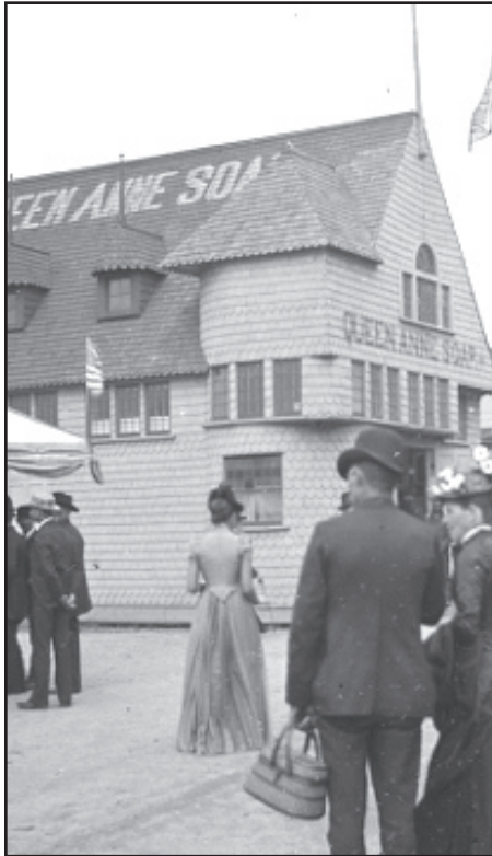
The Queen Anne Soap building in Detroit
