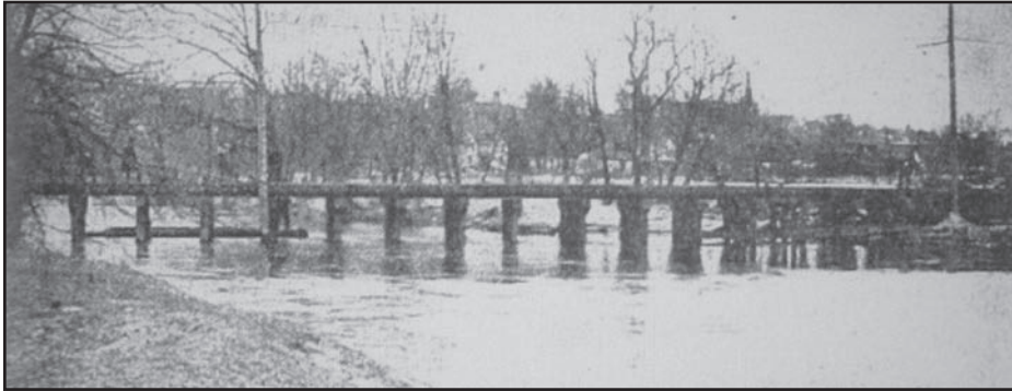
Above: Ypsilanti's 1918 bridge set new records for the industry. Right: Pile drivers c. 1918
