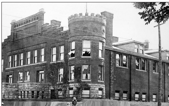
The exterior of the gymnasium was of brick with trimmings of Berea stone and its architecture was medieval in style. The building was divided into a south half for men and a north half for women.
